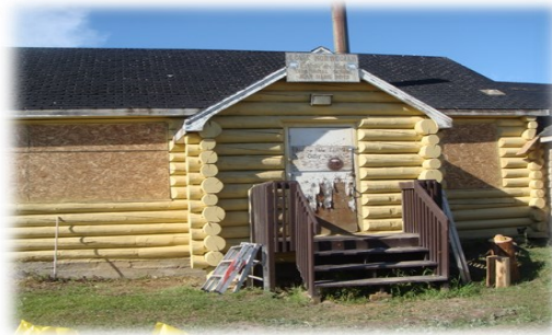
Right: the log school after log renovation in summer of 2015.
